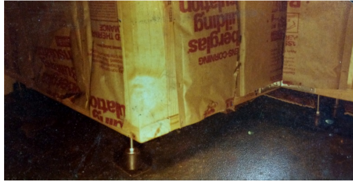
Figure 4. Walls shown floating on neoprene isolators
