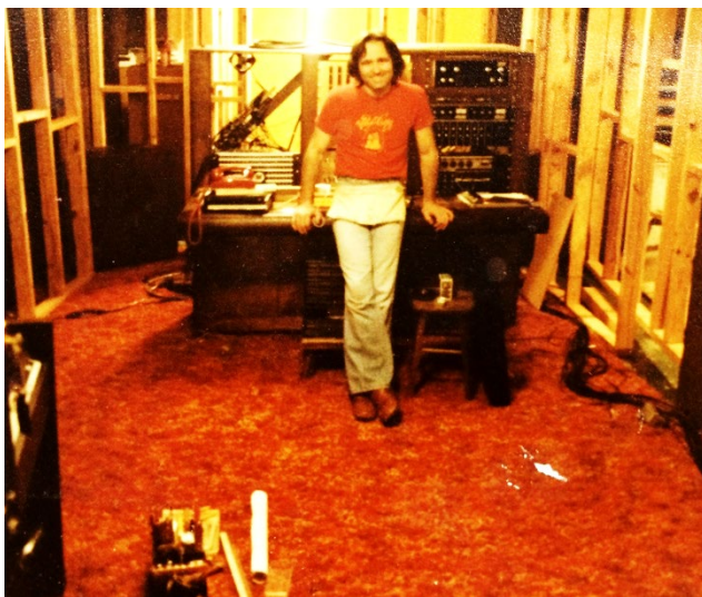
Figure 5. New studio construction and dismantling the old vertical console
