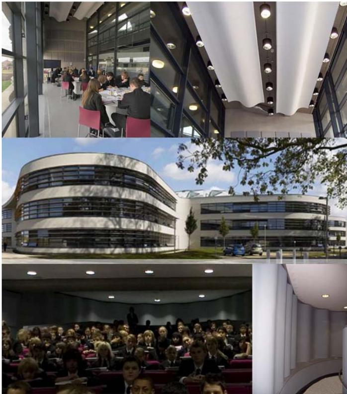
Figure 4. Collage of images at the Thomas Deacon Academy in Peterborough, UK. Upper left and right: Ceiling mounted optimized spline in glass reinforced gypsum; Center: Outside photo; Lower left: Lecture hall optimized wavy rear wall; Lower right: Close up of the optimized wavy wall to minimize focusing effects.
